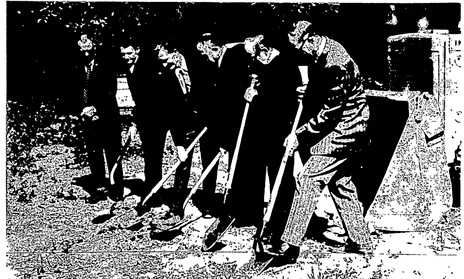
OFFICERS of Waynesville masonic bodies break ground in a ceremony Saturday morning for a new lodge home at the corner of East Marshall and Broadview streets. Paul Bryson, left, chairman, of the building committee, watches as the following five men (listed from the left) break ground: C. E. Morris,
